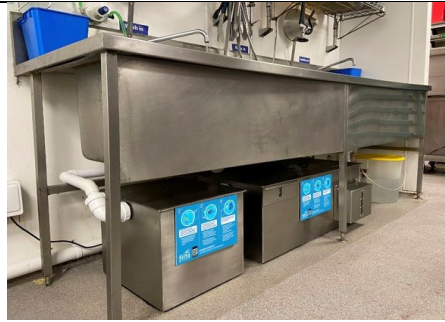
Image 2: The FiltaFOG Cyclone is currently the grease separator with the highest rate of grease recovery – here two units in combination
