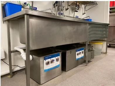
Image 4: Two FiltaFOG Cyclone grease recovery units in combination
